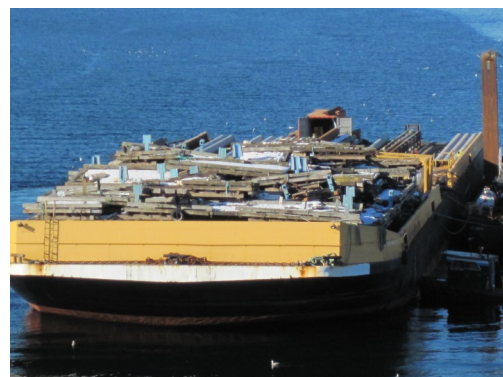
Barge removing docks in ANB Harbor, Sitka, Alaska. Photo: Marnie Chapman
